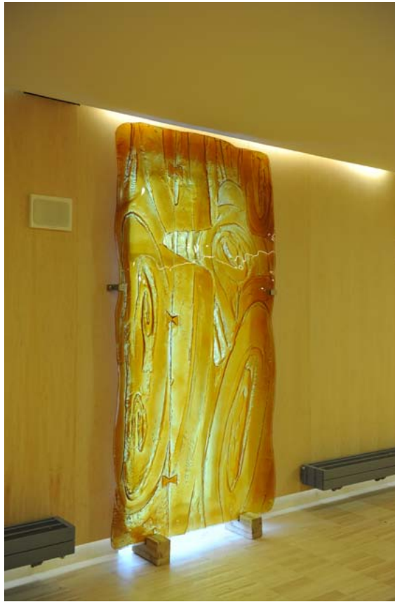
Fig.36. Wooden blocks and metal fixings © Tomasz Urbanowicz
