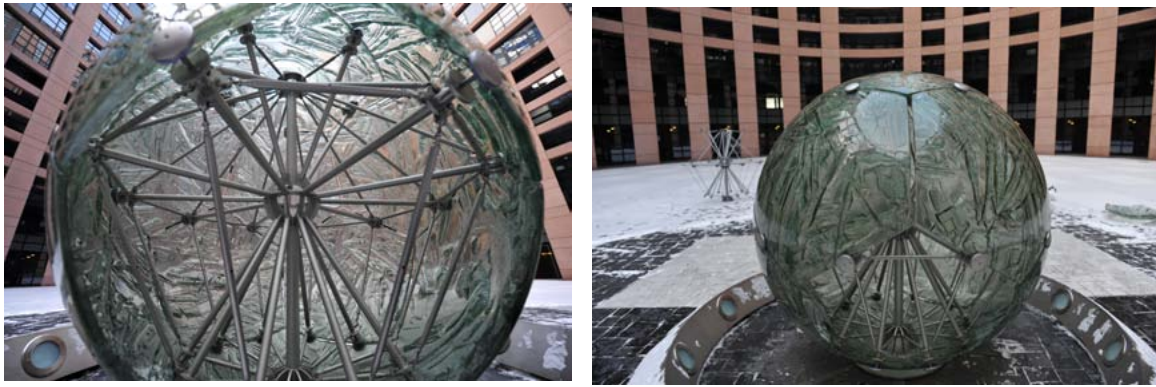
Fig.25. Left - the new frame with some glass attached Right - one more section of glass to attach with the old frame in the background © Tomasz Urbanowicz
