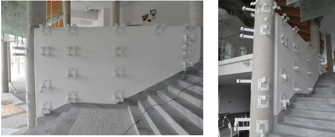
Fig.21. Images of the specially designed fixings for the wall and column panels at the Podlasie Opera and Philharmonic European Arts Centre © Tomasz Urbanowicz
