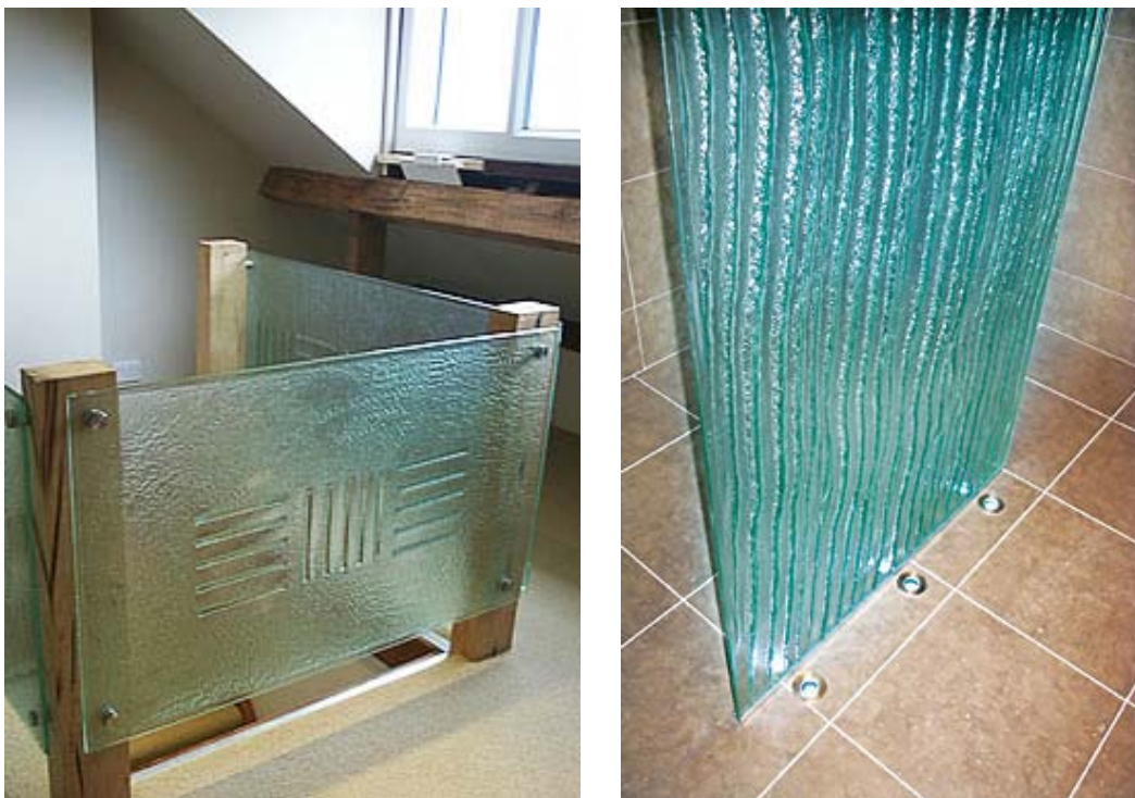
Fig.13. Installations using typical commercial fixings for a balustrade and shower cubicle by Hot Glass Design © Hot Glass Design
